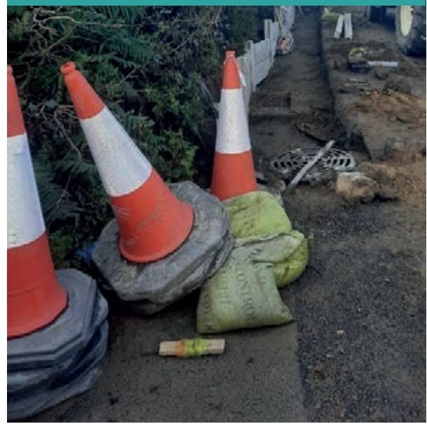
Surface Water Drainage Remediation
