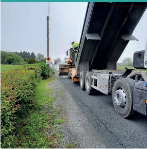
Surface Dressing Operation
