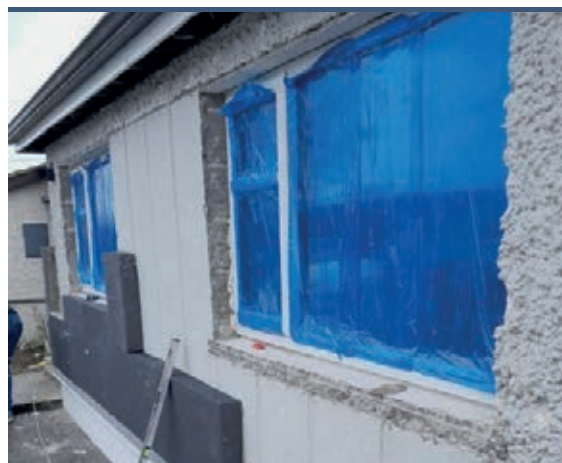
External Insulation being fitted under the EERP Programme
