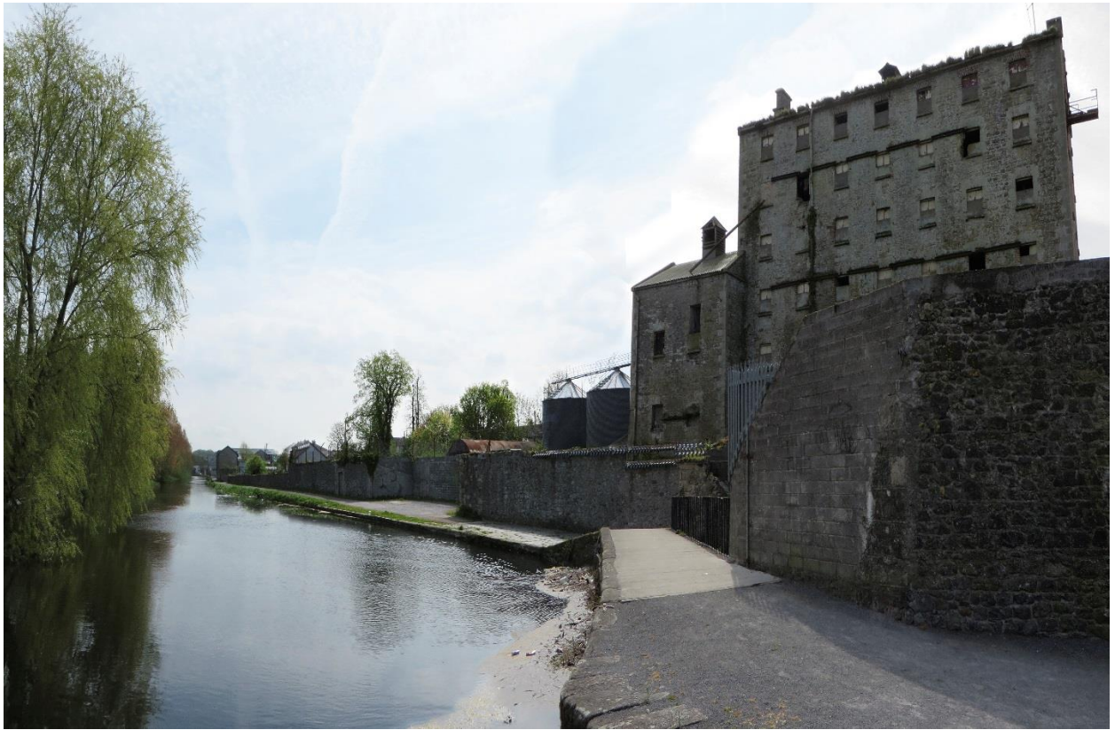
Fig 7 View of Canal Front
