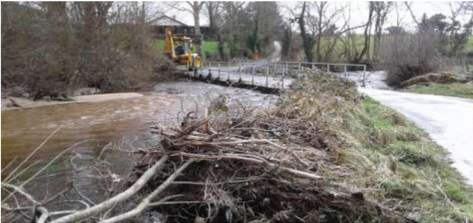
*Clearing Debris from bridge for structural assessment.*
