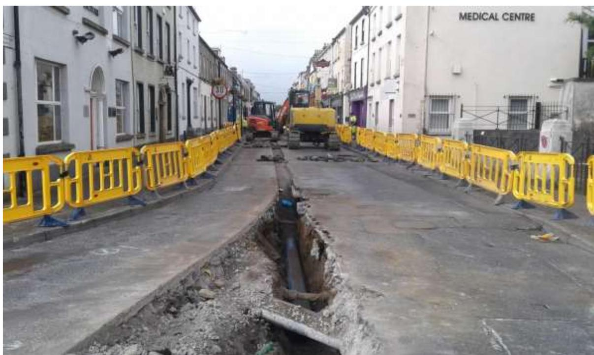
***New Watermain Laying – Threading the needle – Dublin Street. July 2019***
