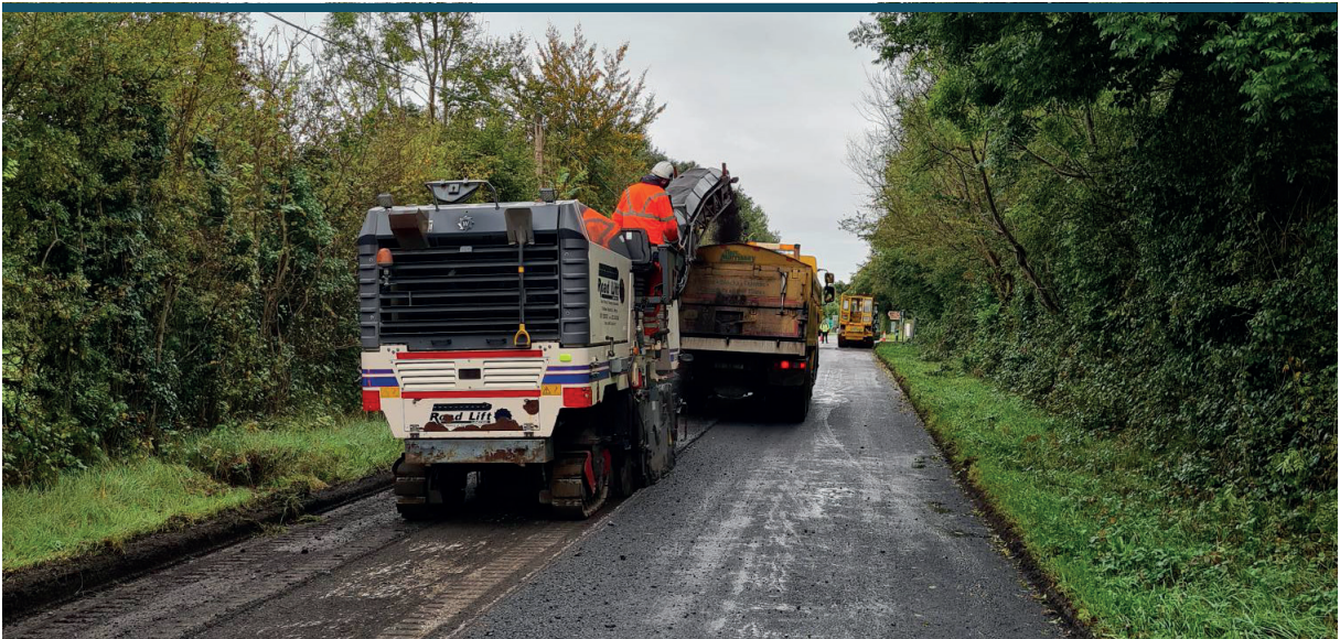
Oibreacha athdromchlaithe ar an N81 ag Crois Mhic Craith
