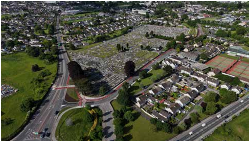
Dublin Road Pedestrian & Cycle Scheme
