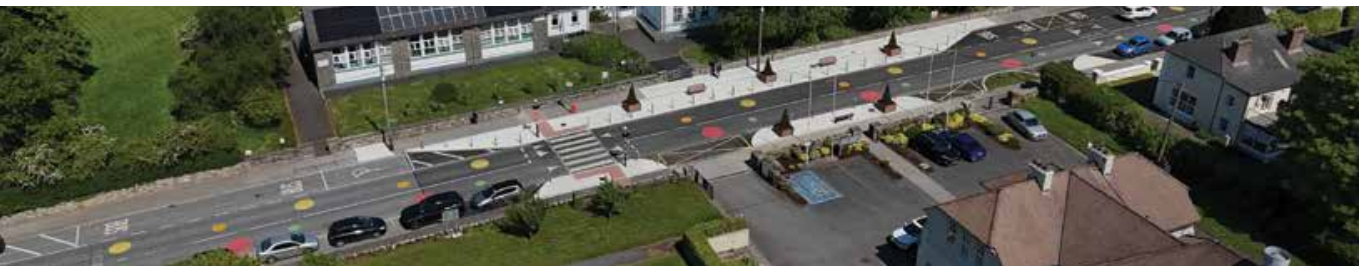
Completed Safe Routes to School Scheme at St. Brigid's National School, Station Road, Bagenalstown
