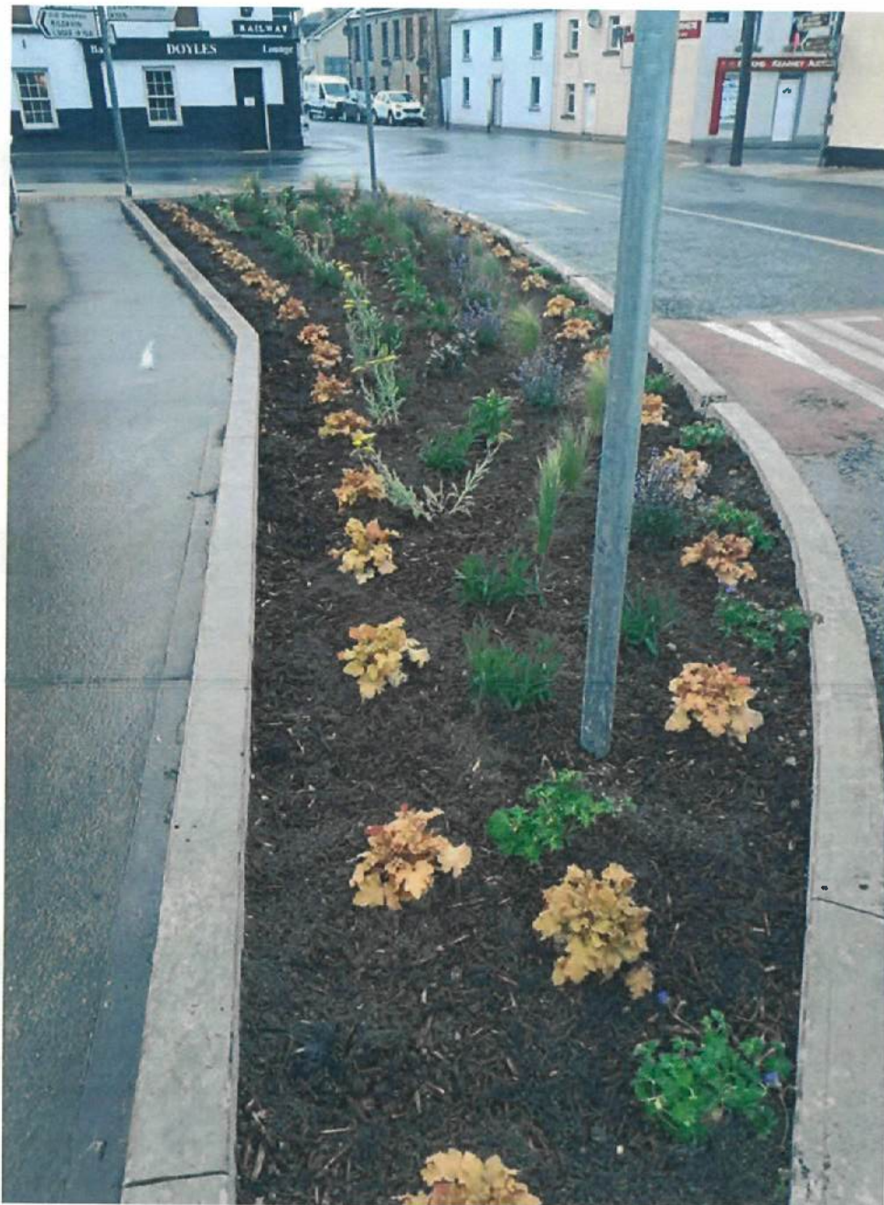
Figure 2. Junction improvement at PIA 5 – Church Street Kilree Moving traffic flow further away from neighbouring properties.
