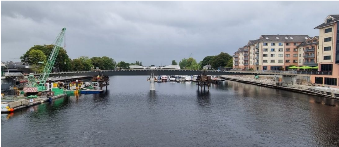
Figure 9 - Dublin Galway Greenway: Athlone Bridge Lift (September 2022)
