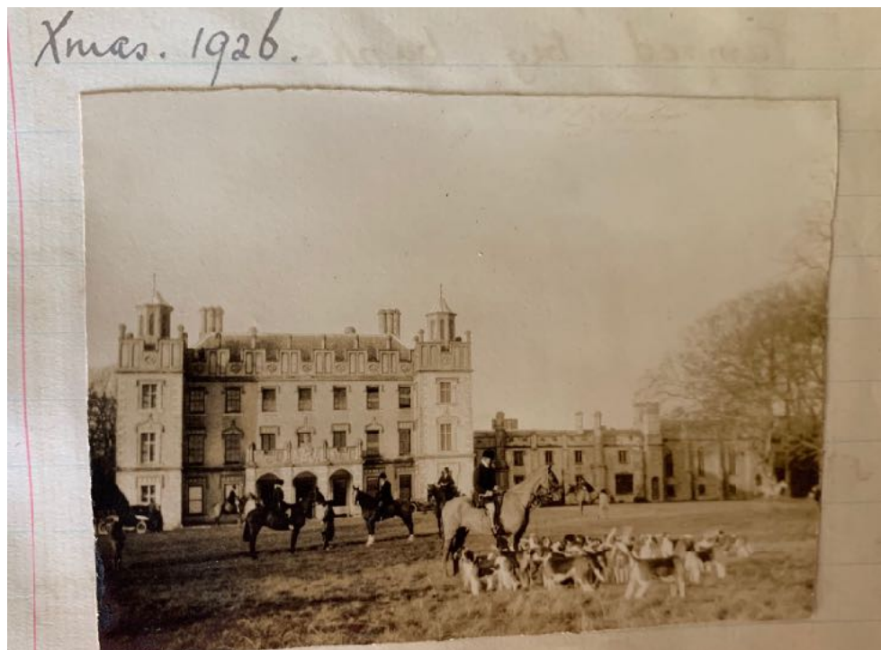
1926 No wall in front of house
