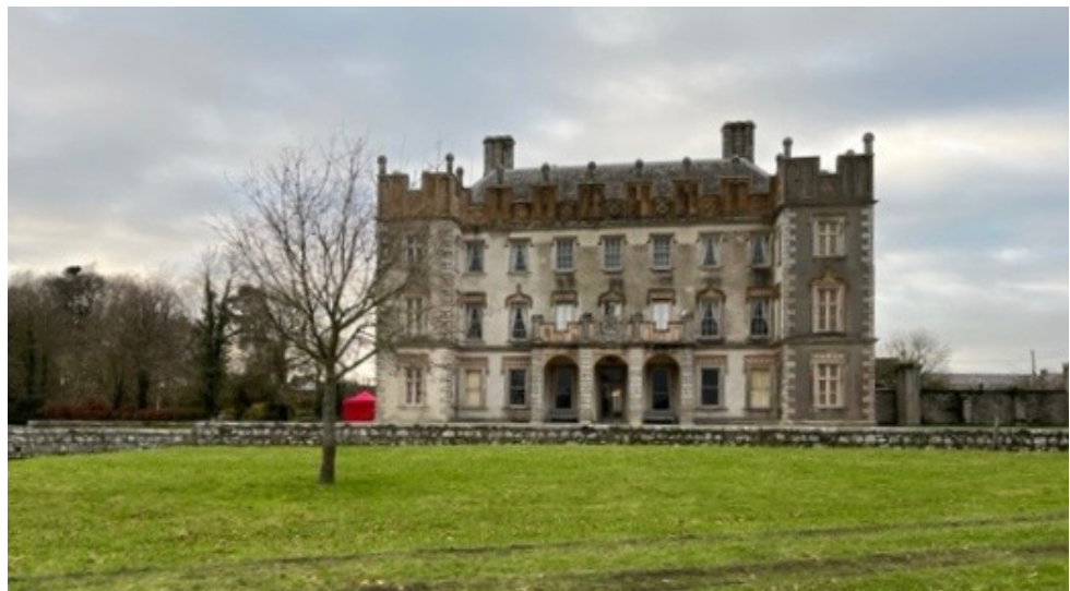
Present frontage with wall between parkland and house
