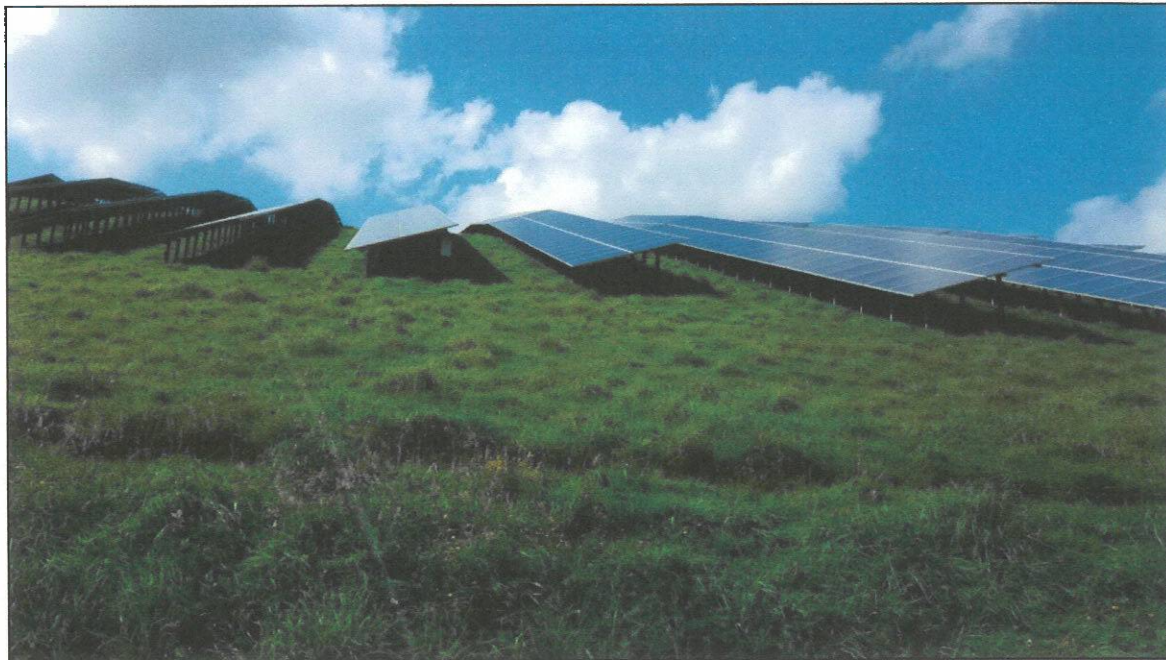
Insert 2-2: Photograph of the Ground Beneath the Solar PV Panels at the Trequite Site
