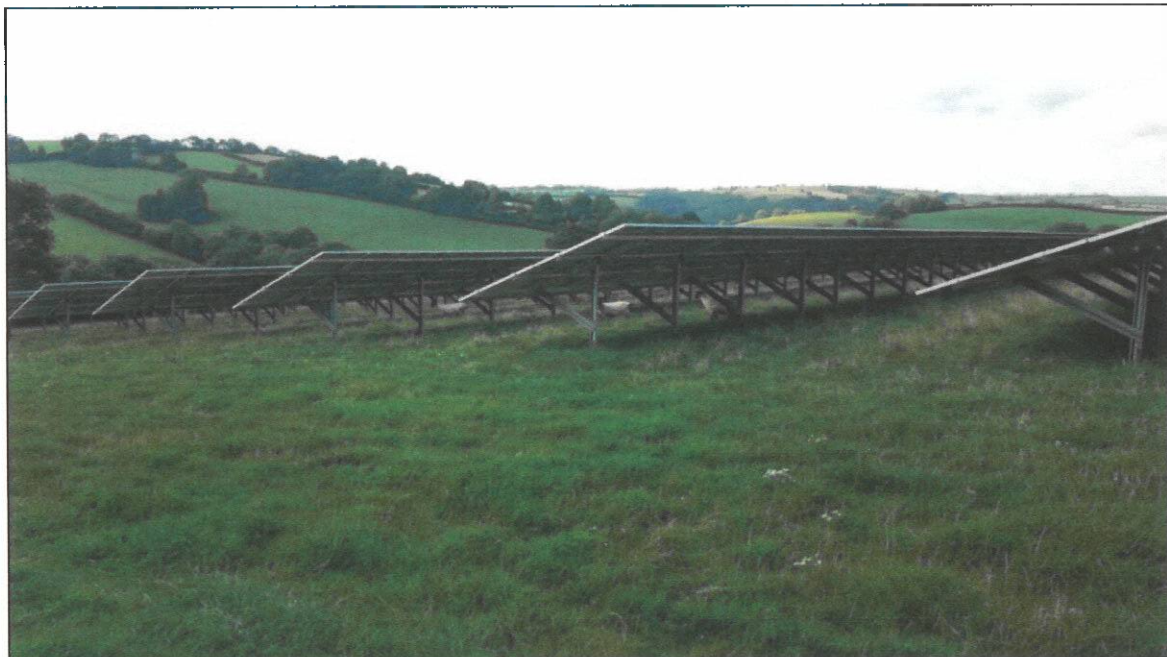
Insert 2-3: Photographs of the Ground Beneath the Solar PV Panels at the Trewidland Site
