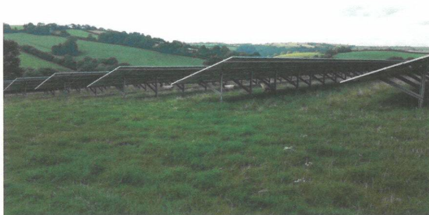
Trewidland – Photographs of the ground beneath the panels at this site that has been in operation since 2013.
