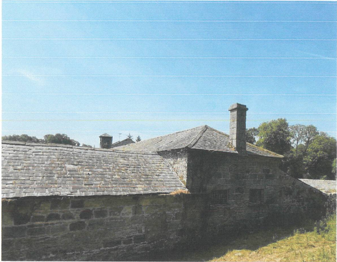
Fig 8 Gable of the building with chimney. Lower building in the foreground is not part of the present works.
