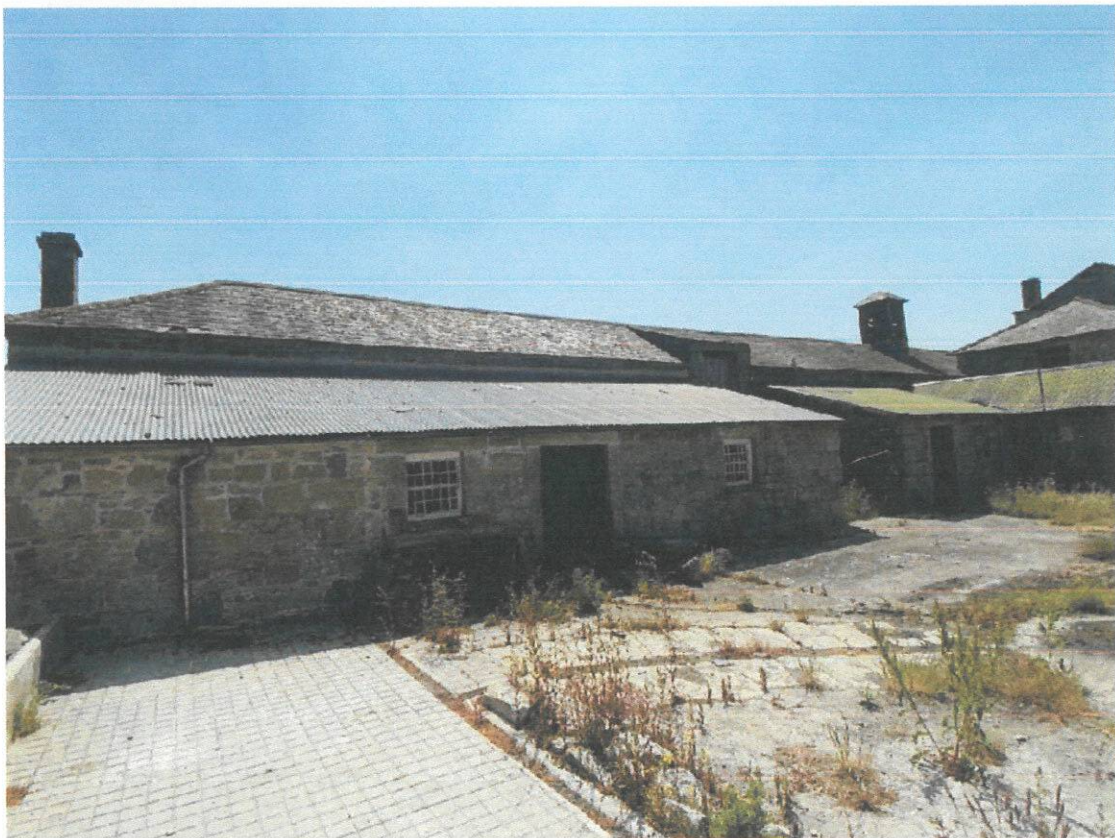
Fig 7 Rear elevation of the building. Lean-to buildings on this side are not part of the present works
