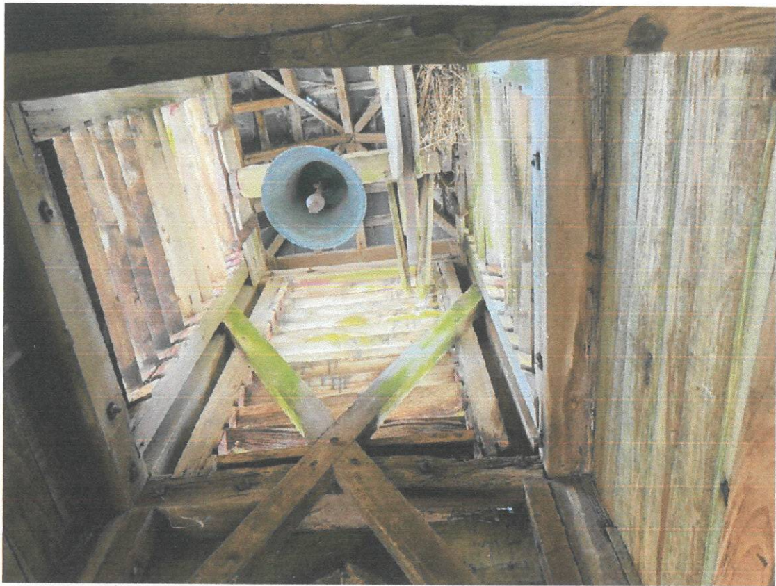
Fig 10 Interior of belfry
