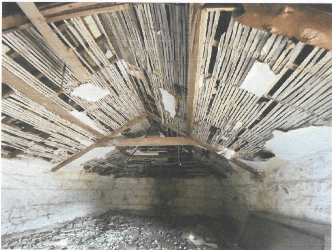
Fig 11 Interior of roof in further section including the hip and the base of the chimney. It is not proposed to re-instate the lath and plaster at this stage. It will be left in place as far as possible.
