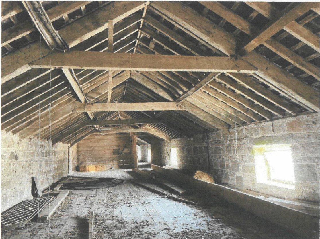
Fig 9 Interior of roof to be re-slatted
