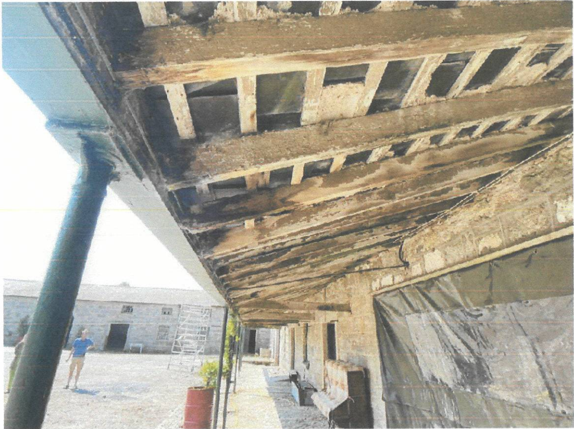
Fig 6 Underside of lean-to.
