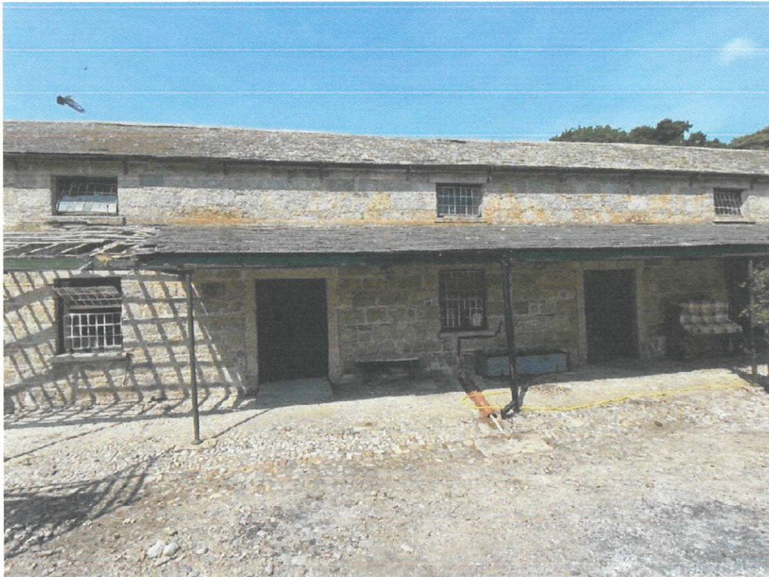
Fig 4 Front elevation of two storey building with lean-to shelter over the doors. Cast iron window glazing can be seen. Collapsed section of lean-to to the left.
