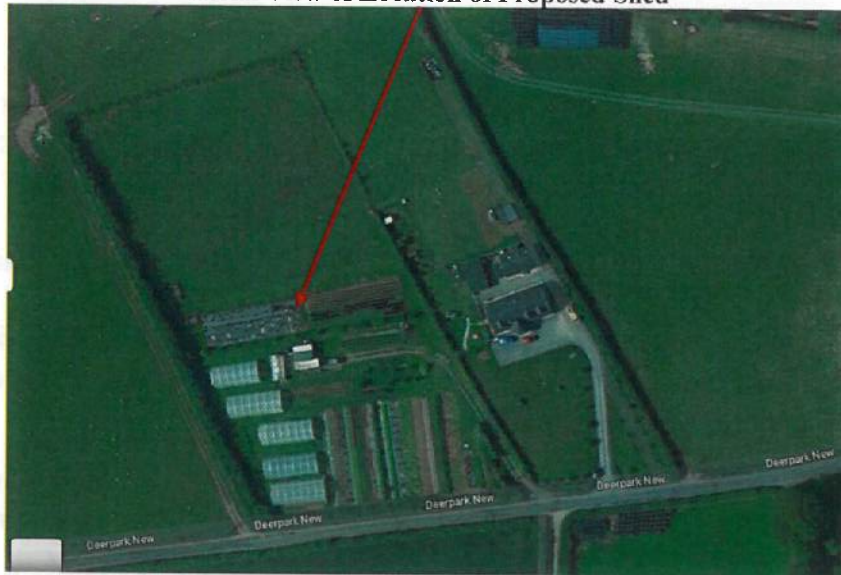
Aerial View of Location of Proposed Shed
