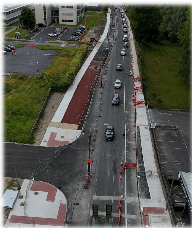
Active Travel Pathfinder - Carlow to SETU Pedestrian & Cycle Scheme under construction
