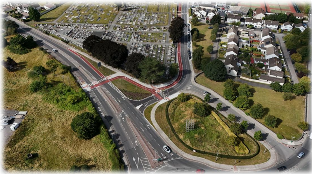
Dublin Road Pedestrian & Cycle Scheme, Carlow Town
